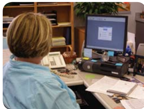
New Valcom "state of the art" digital intercom system (operated by the school office computer) was installed at Belvidere Elementary School in December, 2007.
